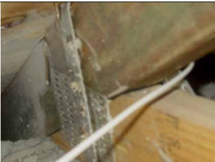
Roof to wall attachment
