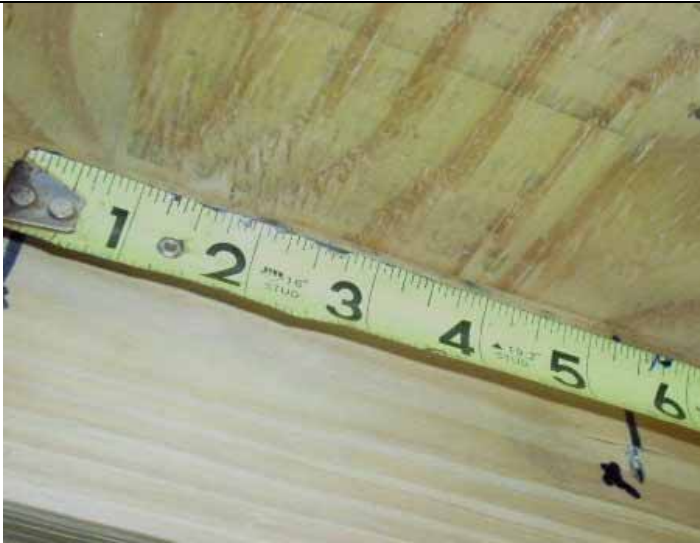
Roof deck attachment
