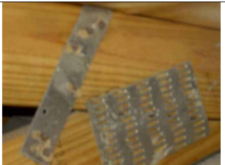
Roof to wall attachment
